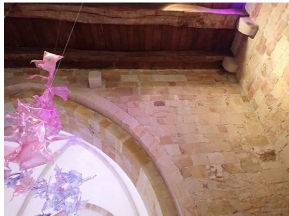
Westwand FG, Turm
