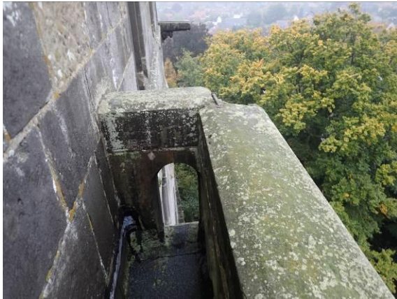
Obergurt Balustrade West
